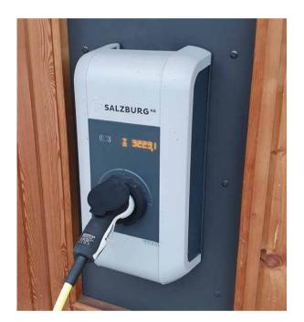
cycle of the signal (Pulse Width Modulation, or PWM) tells the EV the maximum current the EV can draw per phase. A duty cycle of 10% for example, means that the EV can draw 6 amperes at most, depending on the maximum cable capacity.
