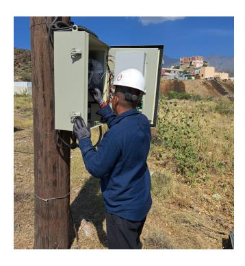
To make maintenance of electrical network assets along the power lines easier and less time-consuming, Al-Ojaimi connected the equipment with the control centers over the public mobile phone network.
